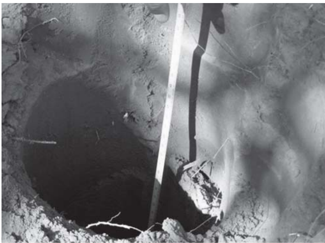
Figure 4 – Trench for collection of sub grade material (Photo: Wallen Medrado).
