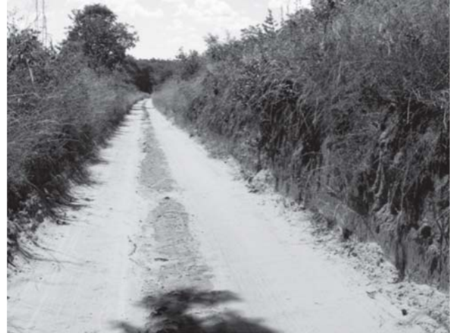
Figure 5 – General view of the road. Cut section. (Photo: Wallen Medrado).
